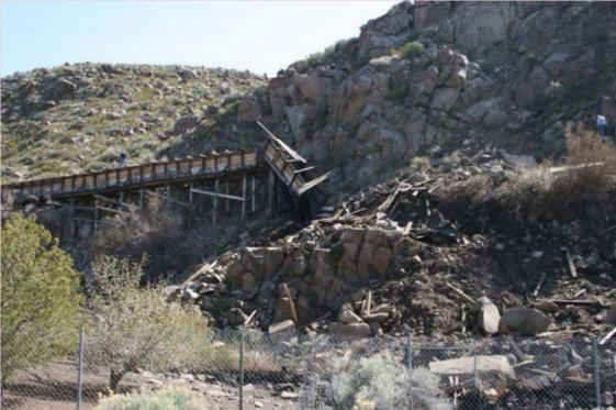
Rock fall damage to water flume (Nevada Bureau of Mines and Geology, University of Nevada, Reno; dePolo 2008)
