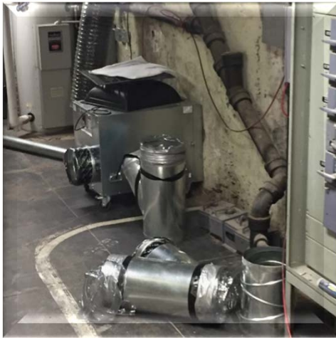
Decommissioned Radon System
